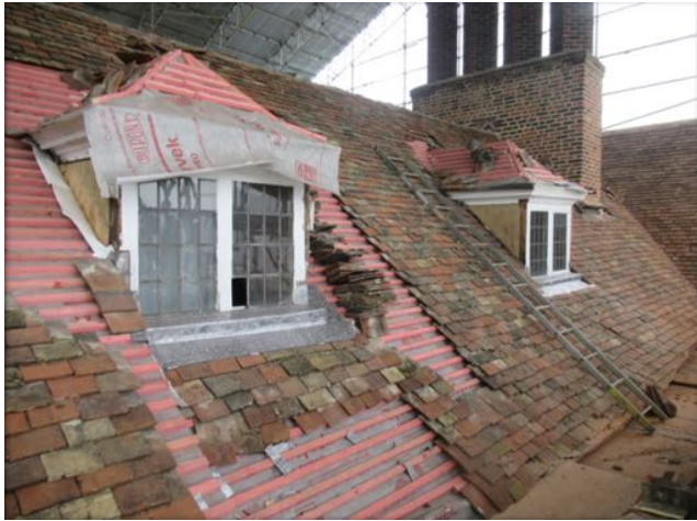
Refurbishment of dormer windows on eastern roof, February 2021
