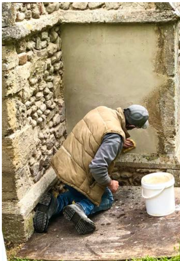
Colin Debenham of Hibbitt Masonry rendering the repaired buttresses (photo: Chis Baldwin)
