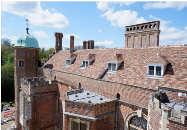
Completion of principal clay-tile roof, May 2021
