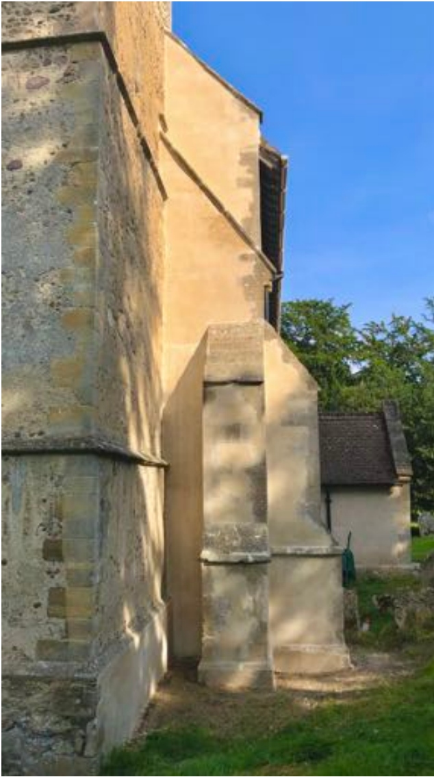
Repairs to the SW buttress
